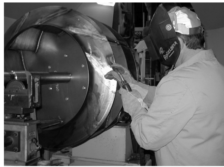
Welding balance plates to a centrifugal wheel prior to painting. (Shown on dynamic balancing stand)
