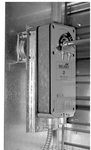
Damper with actuator mounted internally
