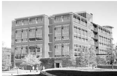
Radio Shack, Corporate Headquarters, Fort Worth Texas
